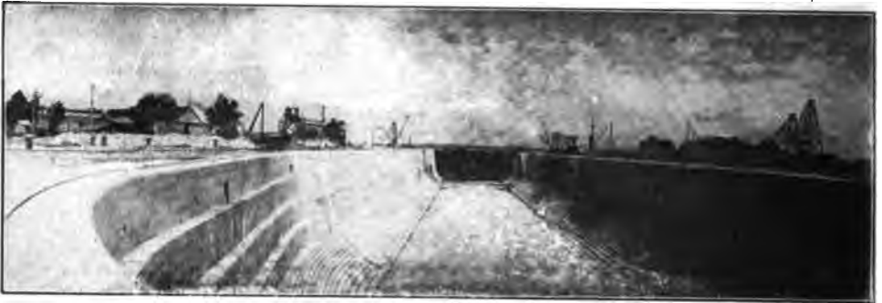
U. S. GOVERNMENT DRY DOCK AT NAVAL STATION AT CHARLESTON, CONSTRUCTED OF WINNSBORO GRANITE.
